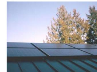
Another row of PV panels was added below this array, for a total of 3200 watts, in this grid-tied battery backed up solar electric system in Sequim, WA.
