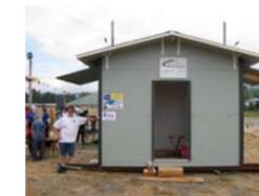
This building, a pop-up, can be assembled and in working order in a half hour. Intended for Emergency Management, it is quickly deployable.
