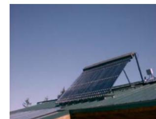
30 evacuated tube solar hot water collector for a preheat system in Sequim. Nearby is 3200 watts of PV power.
