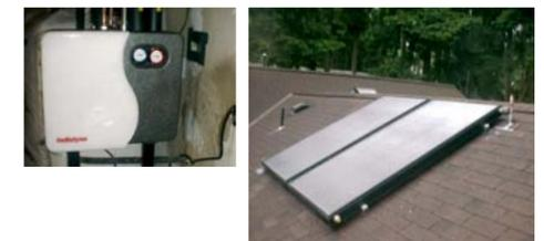
Bainbridge Island is home to this Heliodyne dual flat plate collector system. Heliodyne redesigned their Solar DC pumped external heat exchanger system, opting for a simpler AC pumped system. Works well, providing 80 gallons of preheated domestic hot water.
