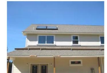
The Heliodyne dual flat plate collector installation went in shortly after this new building was framed and shelled. The preheat system will save hundreds of dollars per year. Port Angeles, WA.
