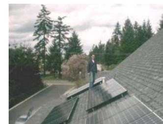
4000 Watts of grid-tied PV and a Heliodyne dual flat plate collector solar hot water preheat system. Bremerton.
