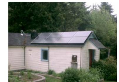
These 1600 Watts perform for a grid-tied battery backed up system west of Port Angeles.
