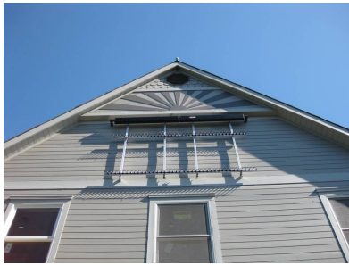
SW Facing Wall (E-Tubes)
