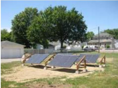
June 6<sup>th</sup> saw an Olympic Energy Systems-developed ground mount solar electric system send electricity to the utility grid in Findlay, Ohio. The University of Findlay installed a two row Tensioned Cable System, the G1, supporting a **2.7 KW** output solar array. The system uses the first production G1.
