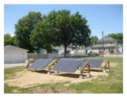
June 6<sup>th</sup> saw an Olympic Energy Systems-developed ground mount solar electric system send electricity to the utility grid in Findlay, Ohio. The University of Findlay installed a two row Tensioned Cable System, the G1, supporting a **2.7 KW** output solar array. The system uses the first production G1.
