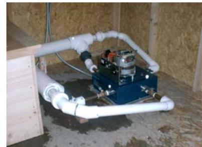
Turbine installed—it's wet because of expected leaks, later fixed with a little silicone gel. The piping moves 150 gallons per minute at 50 psi.
