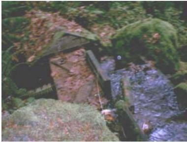
Water Intake at a height of 140 above the powerhouse. Large debris is kept out of the intake by a cover, by a diversion wall, and by the momentum in the flow to the side. The housing acts as a settling tank for sand, silt, and other sediment.
