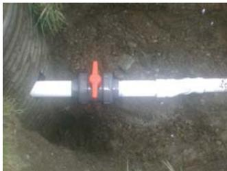
Shut Off Valve on the Penstock, about 45 feet from the Powerhouse. The pipeline still needs to be buried.
