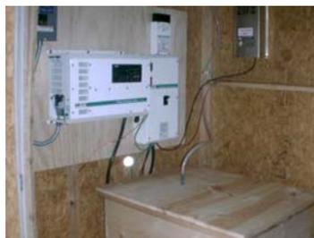
The equipment rack is nearing completion, awaiting a trip to the hardware store for more metal flexible tubing for the wiring to the Air Diversion Load on the far wall.
