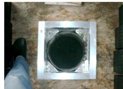
The mounting frame for the turbine assembly. Below is the Tailrace Well. Literally, the design required fitting a square "peg" into a round hole.
