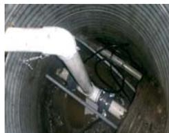
Connection to the main water line. Note the thrust block cable, which counters a force of over 600 pounds.
