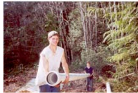
Lower penstock near powerhouse (Crew with Bud Smith)
