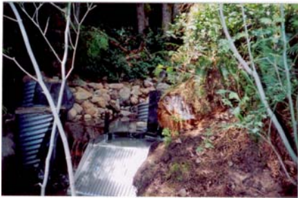
Intake Box at Headworks (soon after installation)
