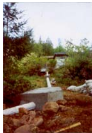
Elevated portion of penstock with jute cover (for UV protection)
