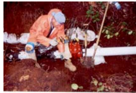
SOV Installation at Headworks (by Geno from Port Townsend)
