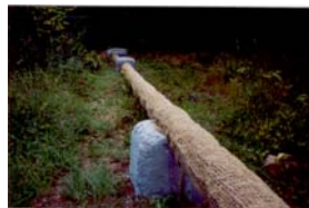
Elevated portion of penstock with jute cover (for UV protection)
