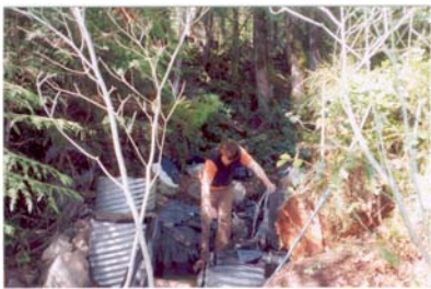
Dominick Smith at Headworks during construction (April 25, 2003)
