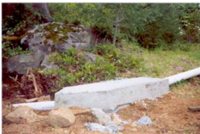
Thrust Block, 45 degrees, near the Powerhouse (100 feet away)
