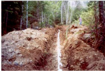
Penstock Installation (C-900 PVC Pipe, buried 2')
